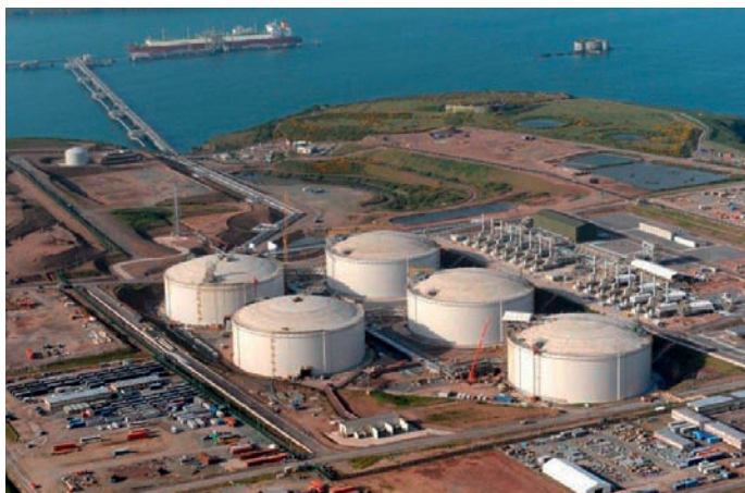
South Hook's re-gasification terminal
