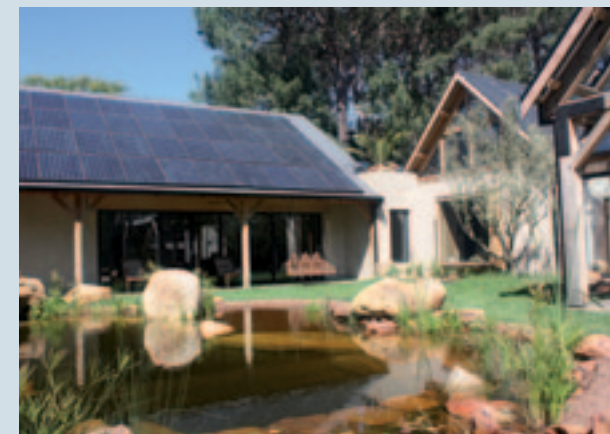
HOUSE GAIA, ROOFTOP INSTALLATION, CAPE TOWN
